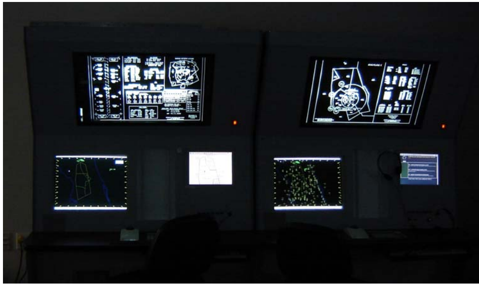
Figure 9. Two ATC Radar Room Workstations
