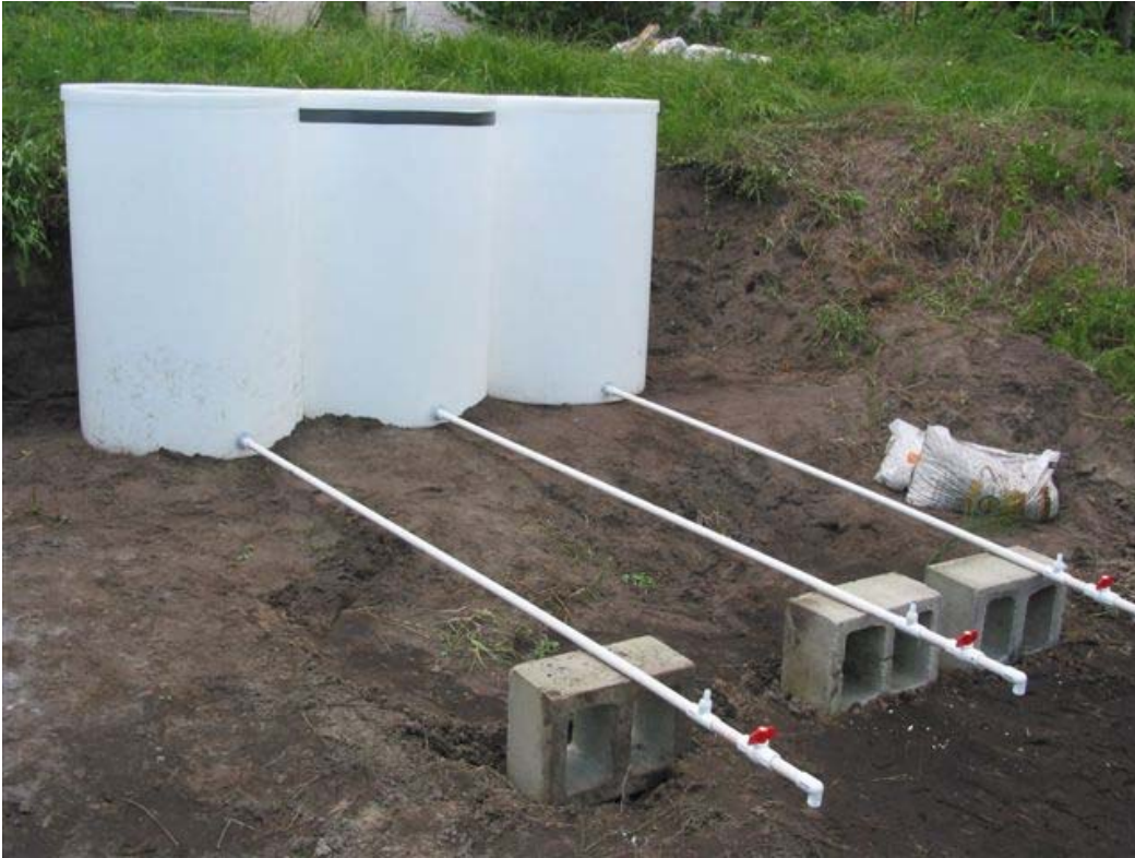
Figure 8: Test Tank Construction in Progress
