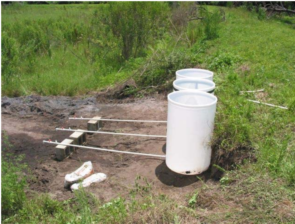
Figure 7: Test Tank Construction in Progress
