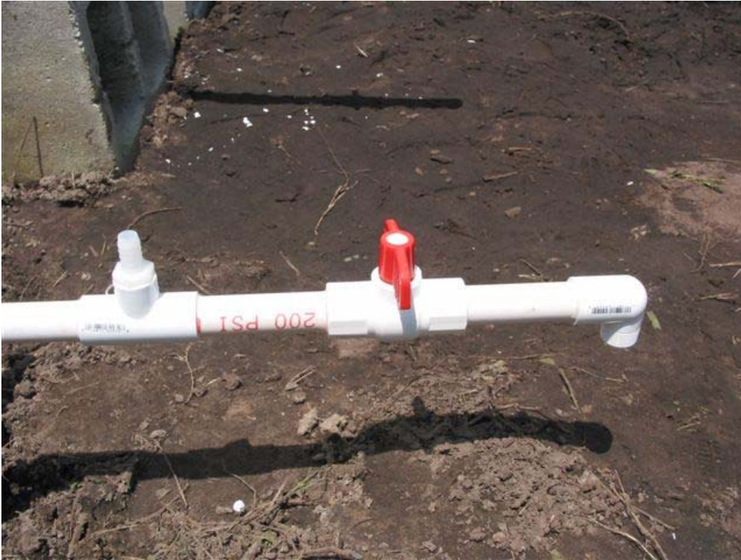
Figure 9: Valve Assembly Details
