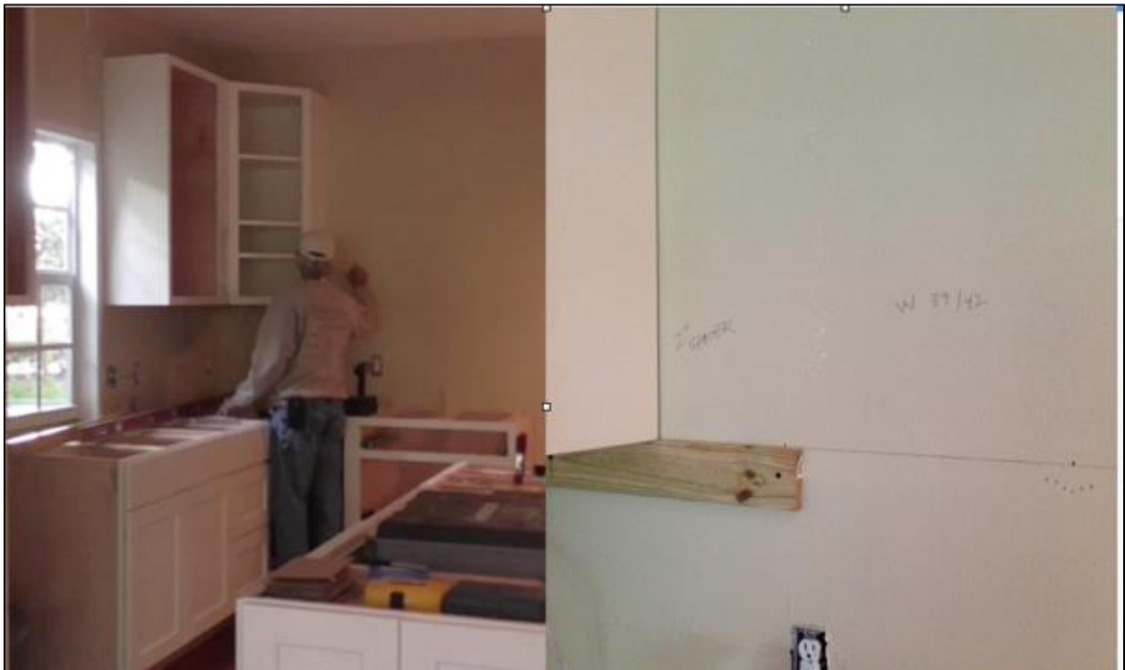
Figure 13: Ned transfers measurements from the CAD drawing to the wall prior to installing a cabinet piece.
