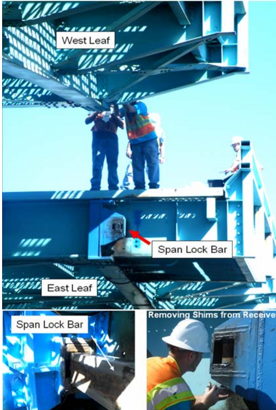
Figure 70. FDOT Contractors Removing Some of the Shims from the SL
