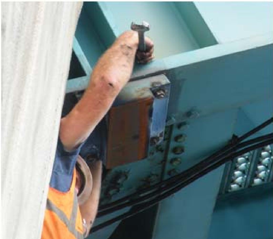
Figure 69. FDOT Contractor Removing Some of the Shims
