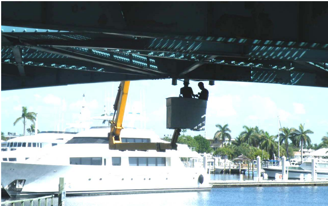
Figure 55: Sensor Installation on Girders
