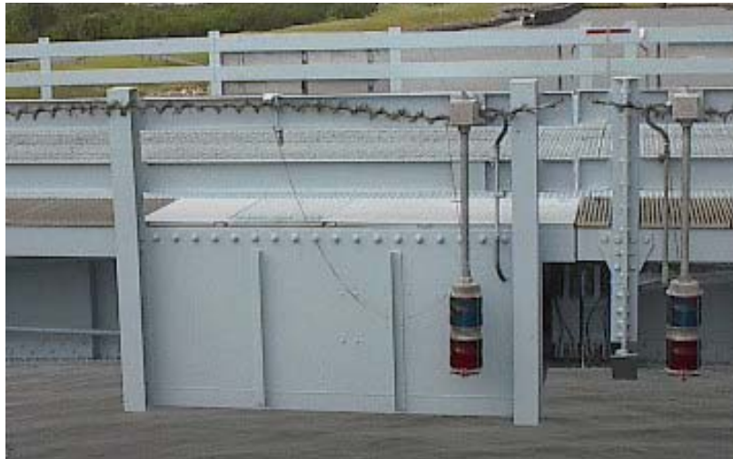
Figure 66. Span Lock Compartment
