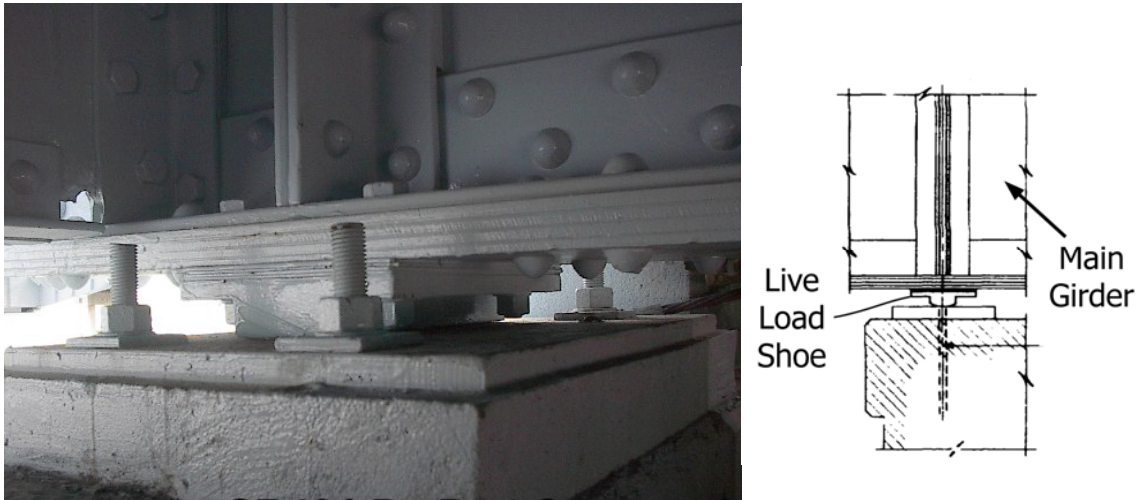
Figure 65. Live load shoe (LLS)
