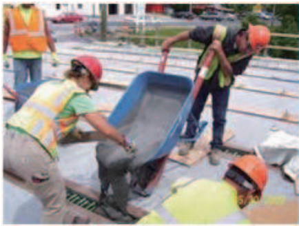
(a) Longitudinal connections cast between deck-bulb-tee girders ([25])
