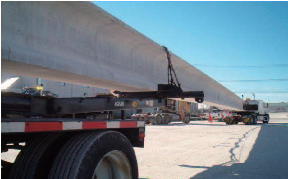
Figure 8: MARS HILL BRIDGE IN WAPELLO COUNTY PHOTO 2
