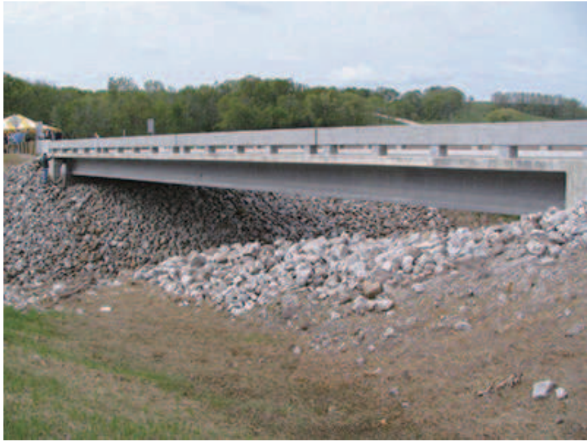
Figure 7: MARS HILL BRIDGE IN WAPELLO COUNTY PHOTO 1
