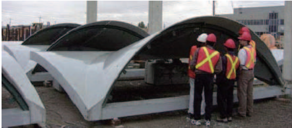
Figure 4: THE SHAWNESSY LIGHT RAIL TRANSIT STATION PHOTO 2
