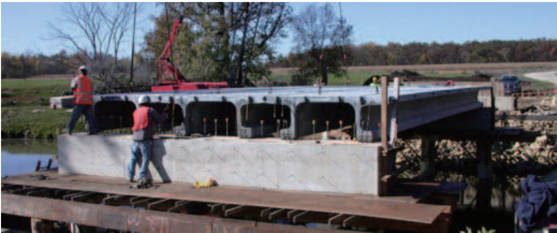
Figure 5: THE JAKWAY PARK BRIDGE PHOTO 1
