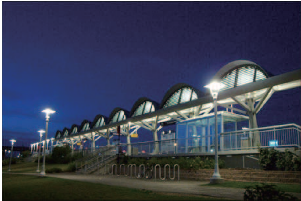
Figure 3: THE SHAWNESSY LIGHT RAIL TRANSIT STATION PHOTO 1
