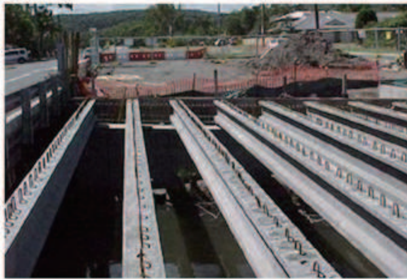
Figure 11: THE SHEPHERDS CREEK DUCTAL BRIDGE PHOTO 1
