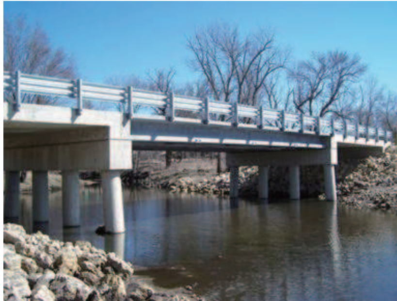
Figure 6: THE JAKWAY PARK BRIDGE PHOTO 2
