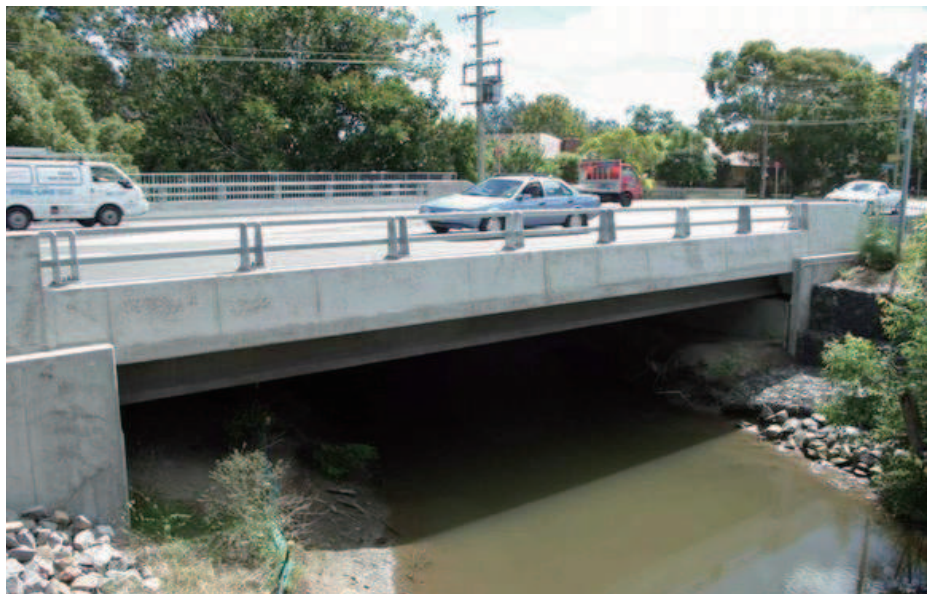
Figure 12: THE SHEPHERDS CREEK DUCTAL BRIDGE PHOTO 2
