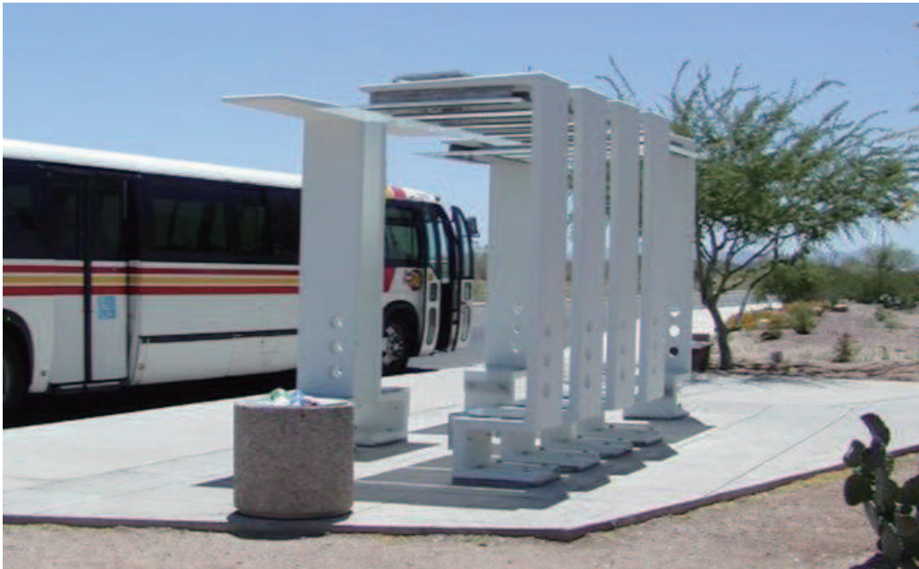
Figure 9: BUS SHELTERS MADE OF UHPC
