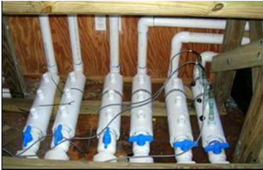
Figure 3.8 The Nadles layout with the probes connected
