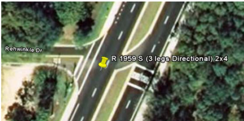
Figure 3-25: Third Aerial Image from “Google Earth” for an Unfamiliar Unsignalized Intersection in Leon County
