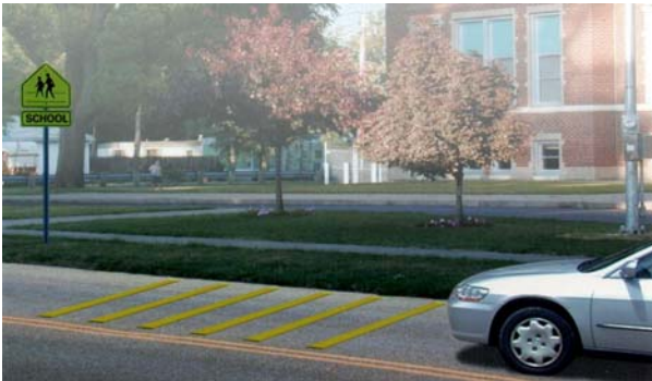
Figure 4-4: Rumble Strips Installation
