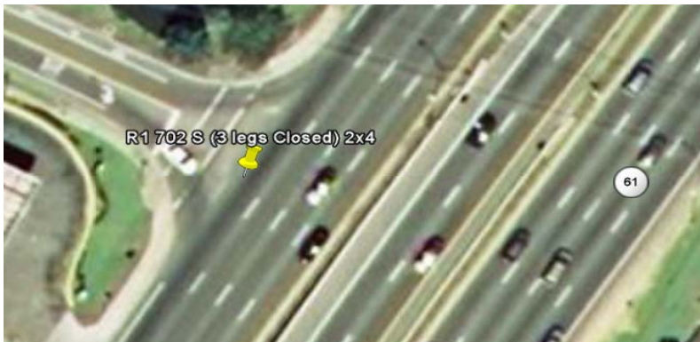
Figure 3-24: Second Aerial Image from “Google Earth” for an Unfamiliar Unsignalized Intersection in Leon County
