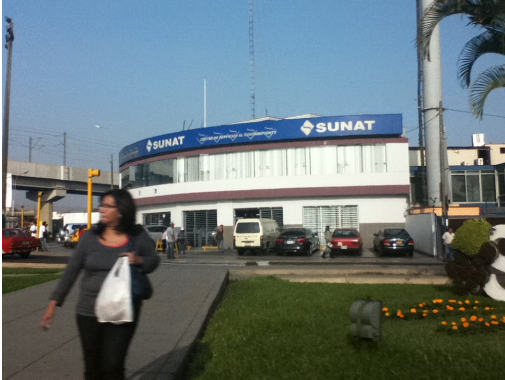
Figure 15: SUNAT Office in Surquillo
