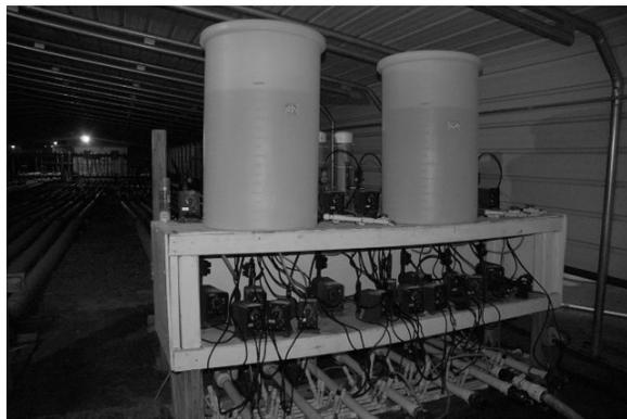
Figure 4.6 Inhibitor tanks and feed pumps
