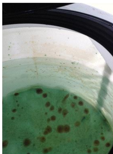
Figure 5-43: Greenish Algae in UF Filtrate Tank
