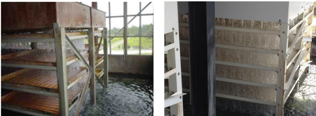
Figure 5-31: Old Tray Aeration System (left) and New Tray Aeration System (Right) at Verna
