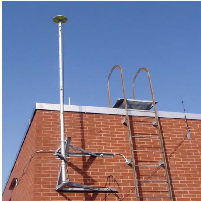
Figure 15: GPS and Radio Antennae for the Base Receiver
