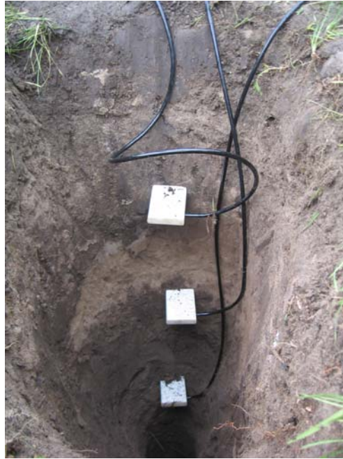
Figure 5: TDR equipment at 1-ft, 2-ft, and 3-ft depths
