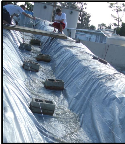
Figure 50: Staggered Configuration after modifications
