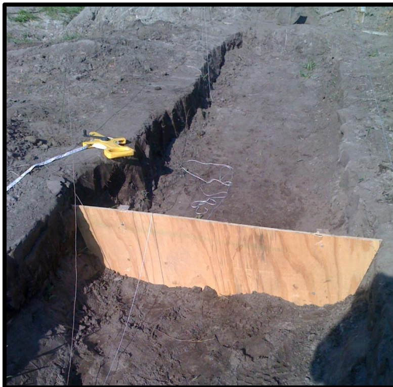
Figure 19: Construction of Hydraulic Jump and Plateau for Collection Mat
