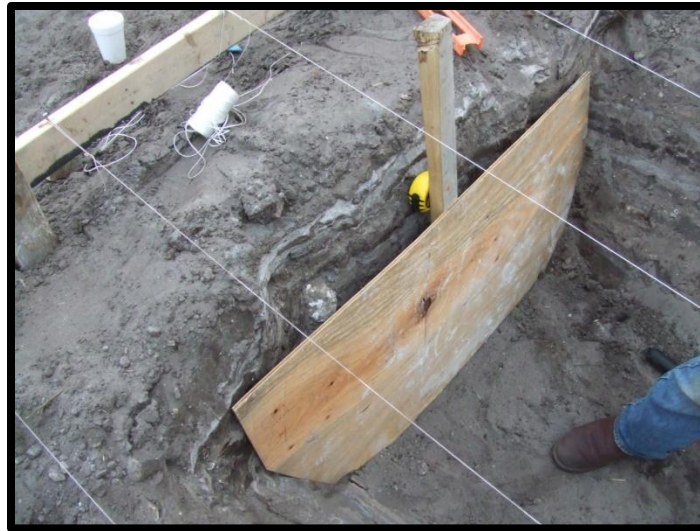
Figure 21: Plywood Cut for 2H:1V Slope
