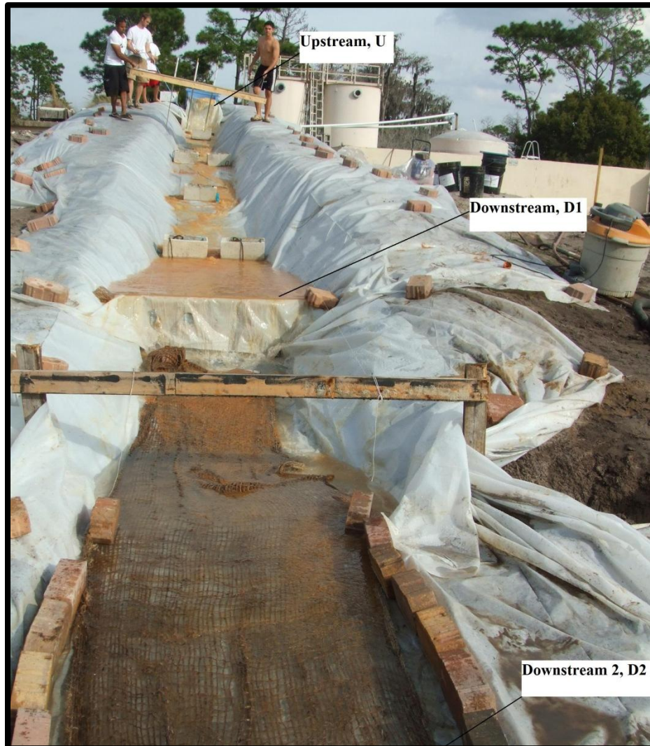
Figure 48: Sample Location for Field-Scale Testing
