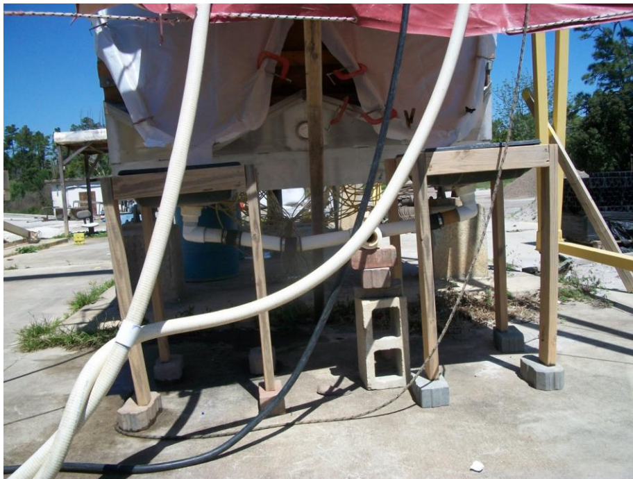
Figure 15: Downstream Collection Troughs and Sinks
