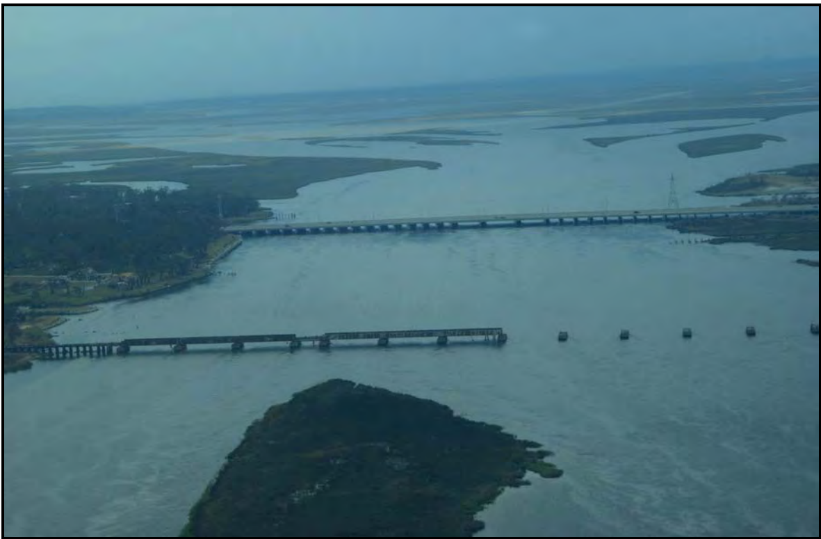
Figure 1.12 Highway 90 (rear) and partially damaged railway (front) on the West Pascagoula River (USGS Center for Coastal & Watershed Studies)
