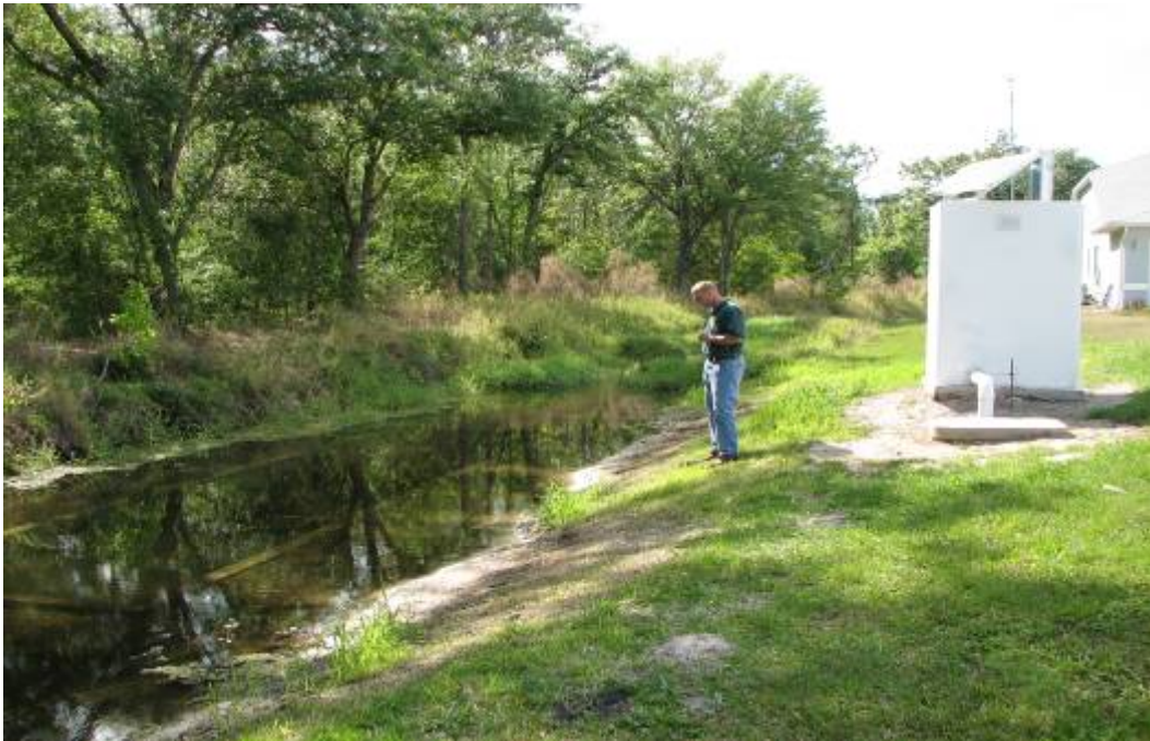
Figure 13: Submerged Concrete Channel
