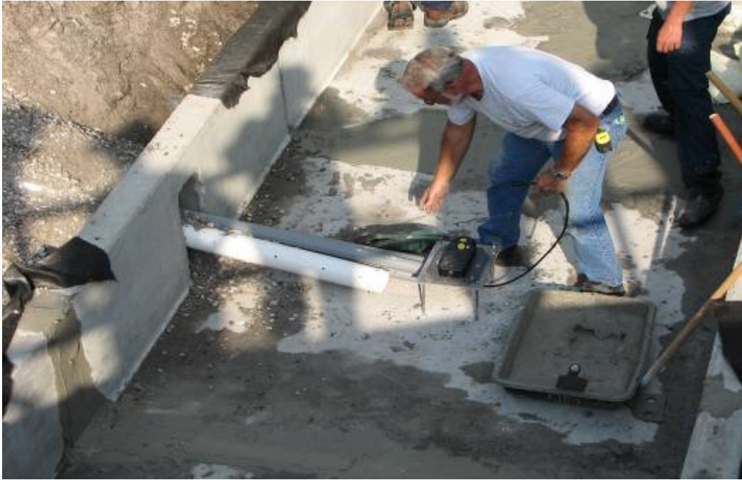
Figure 12: Concrete Channel Equipment Installation
