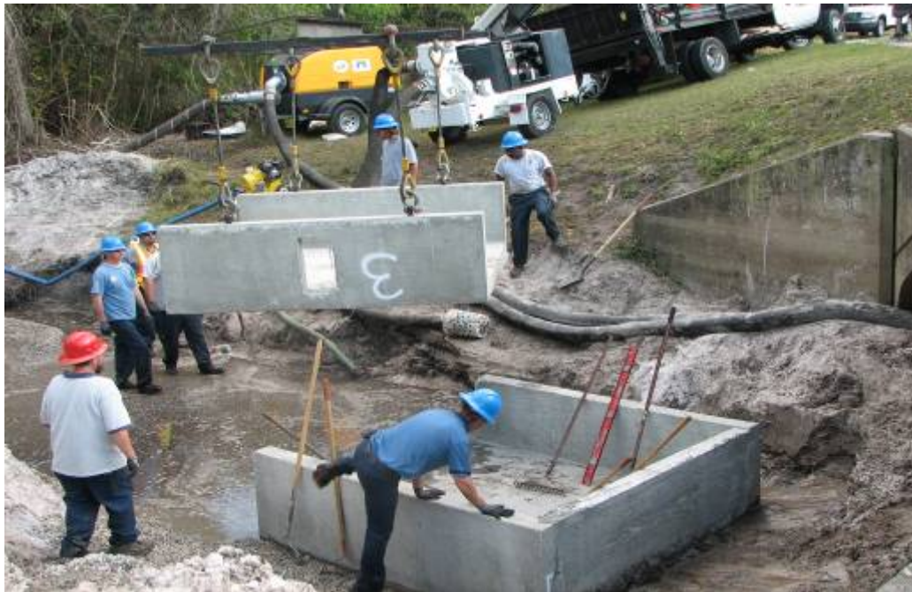
Figure 10: Concrete Box Installation
