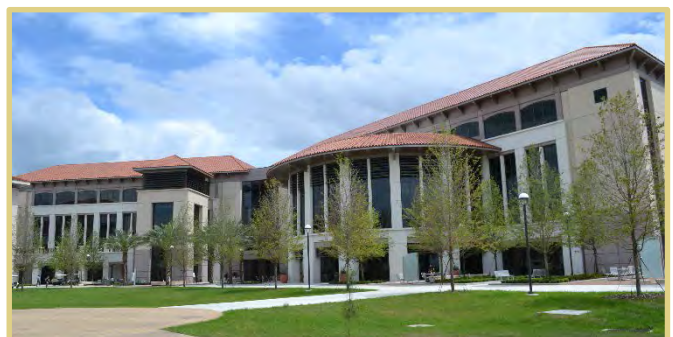
UCF Libraries services are available in the Valencia Osceola Campus Library, building 4, room 4-202
