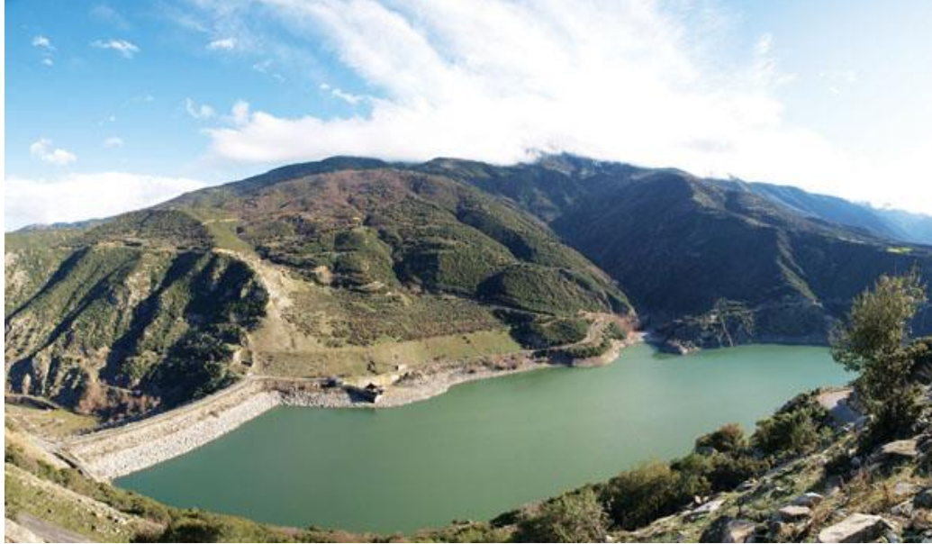
Picture 5.2: Hydropower dam of Polifitos (source: www.portal.tee.gr )
