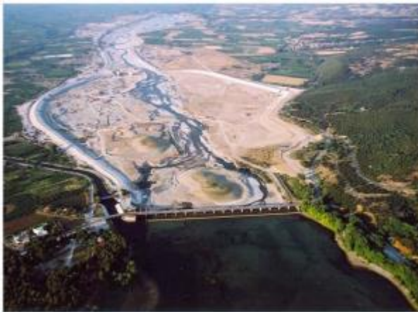
Picture 5.5: Small hydropower plant of Agia Varvara (source: www.portal.tee.gr )
