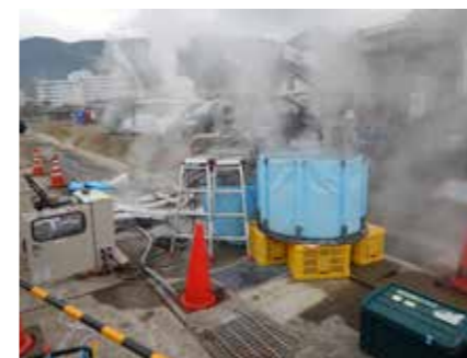
Fig.4 Field test of mechanical descaling.
