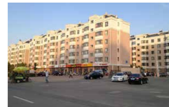
Fig.5 High-rise buildings built in medium and small cities of Inner Mongolia Autonomous Region (2)
