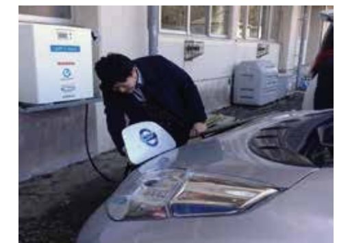
Fig.4 V2H system has been installed in Kazuma elementary school, Ishinomaki city (Task 3)
