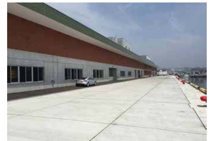
Fig.4 Onahama fish market which was built as reconstruction contracts from the Great East Japan Earthquake Disaster
