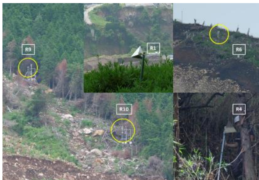
Figure 5.8 Images shown the installed places and orientation of the corner reflectors
