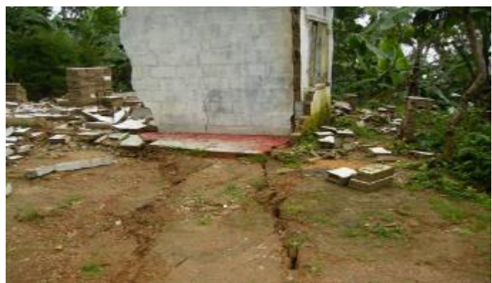
Figure 7.3 affected house during 2007 incident-crack develop arbitrary manner on loose old landslide, Srilanka
