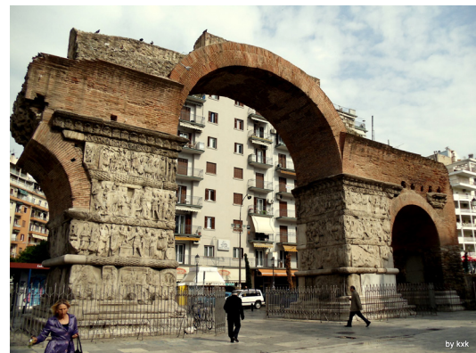
Picture 31: The remains of the arch
