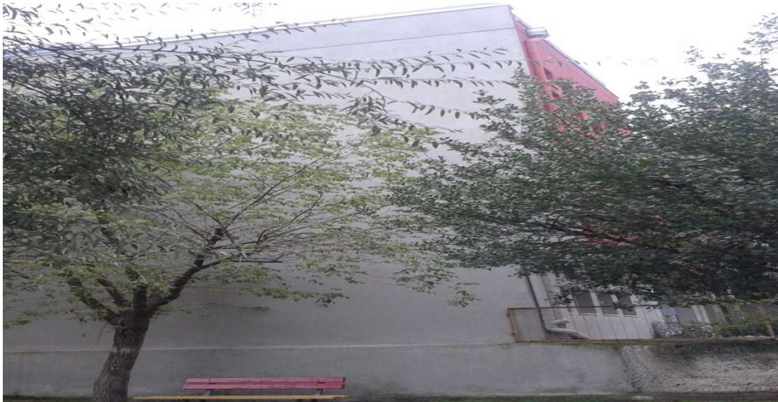
Figures 20: View and facing obstacles of the building
