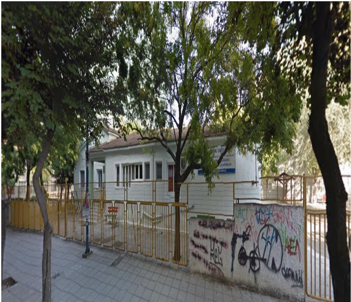
[Energy audit of a kindergarten in Larissa]
