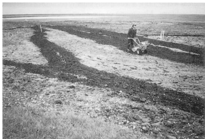
FIG. 10. View of rototilling tundra soil that had been contaminated with crude oil from a spill that occurred in 1969. In 1990, heavily contaminated gravel fill and tundra soil were removed from the site, and tilling was used to promote biodegradation of the remaining hydrocarbons.
