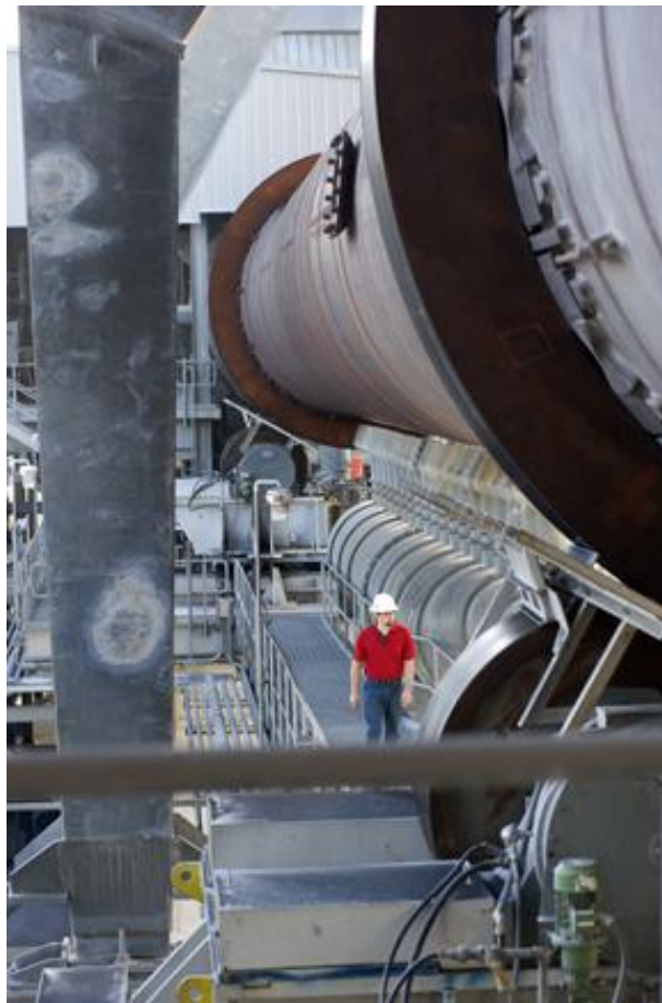
Figure 2: Rotary cement kiln [8]
