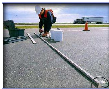
Figure 2–3 Piezoelectric sensors
