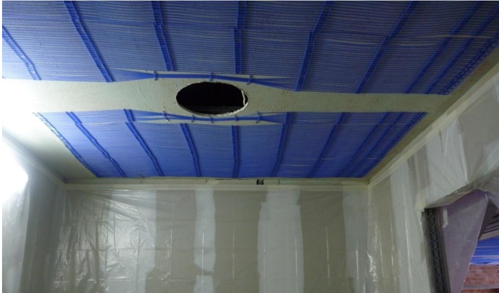
Picture 73: Karo radiative ceiling during installation
