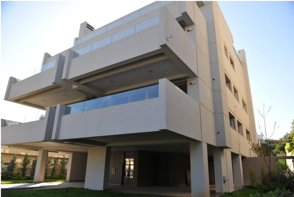
Picture 61: Front view of the residential building under examination
