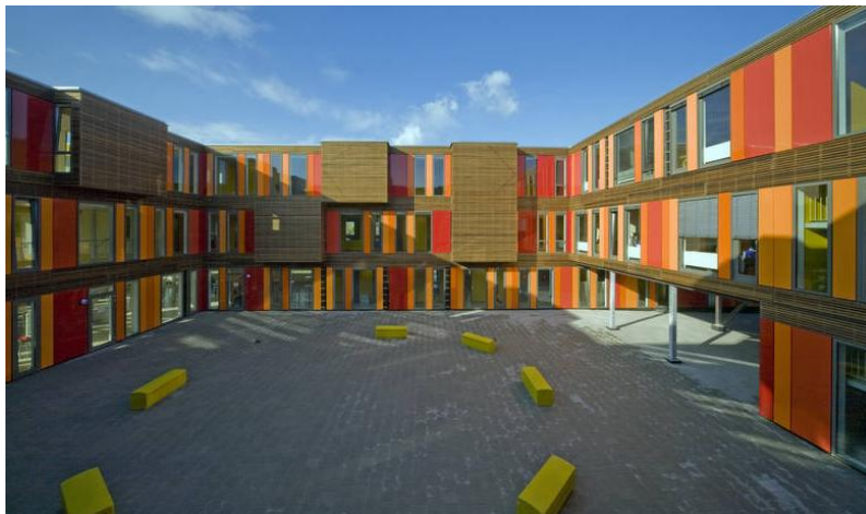
Figure 3.2: 4 th gymnasium, Amsterdam [13]
