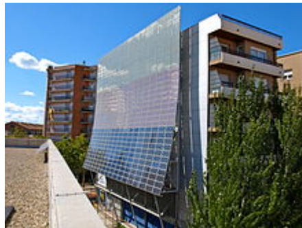
Picture 21: Photovoltaic wall at MNACTEC Terrassa in Spain.
