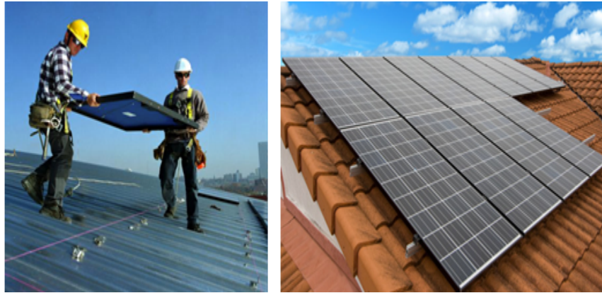
Picture 17: Installation of a residential photovoltaic station.
