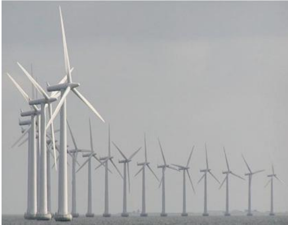
Figure 34: Marine wind turbines off the shores of Copenhagen. Photograph: John Nyberg [32]
