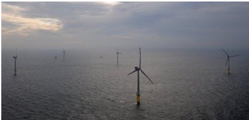
Figure 35: The "Alpha Ventus" wind park, 45 kilometers (28 miles) north of the island of Borkum in the North Sea [33]
