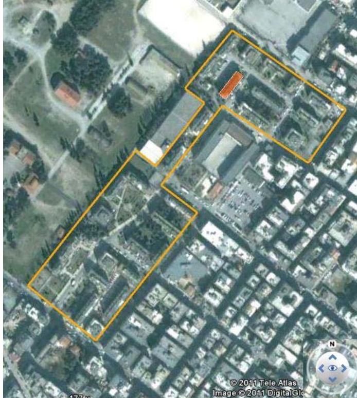
Figure 26: Aerial of the building complex. Marked in color is the representative building under study.
