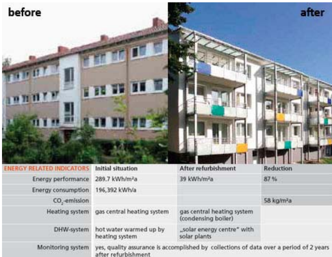
Fig 14: Good practice example of the “Retrofitting of Social Housing” program. The social houses were built in 1955 in Steffensweg, Bremen-Walle and they were refurbished in 2005.
