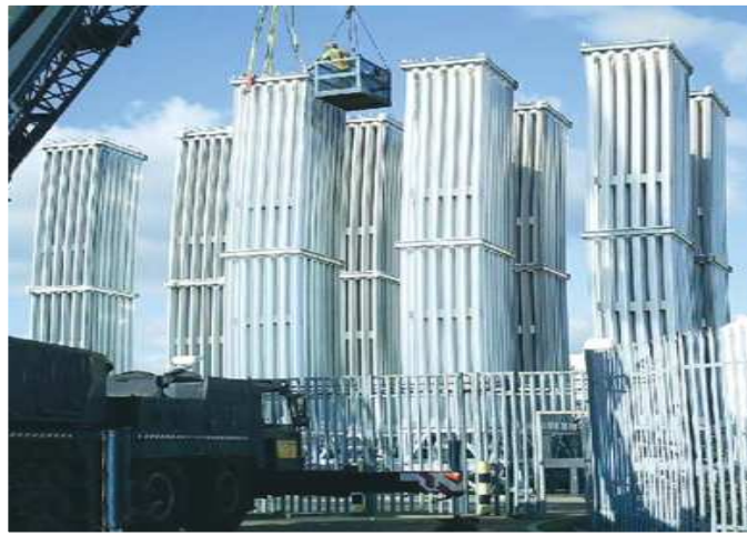
Figure 20: Thermafin™ Supergap™ Ambient Vaporizer. Product of company Thermax Inc.
