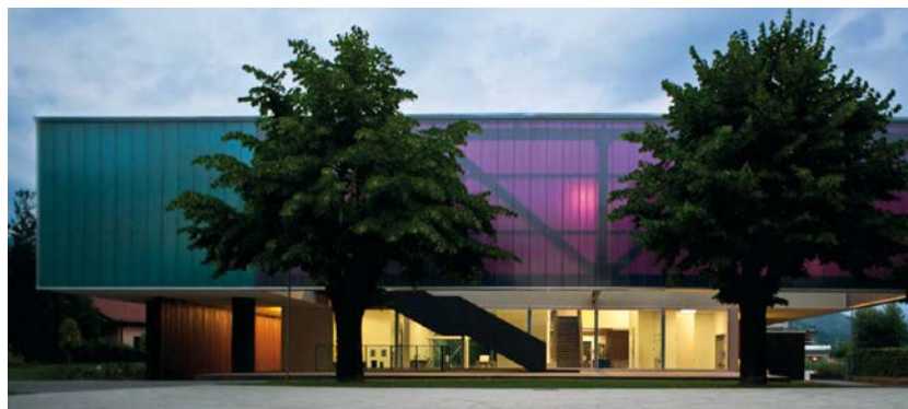
Figure 6: Example of a building clad in PC panels (DAP Studio in Bergamo, Italy). [40]
