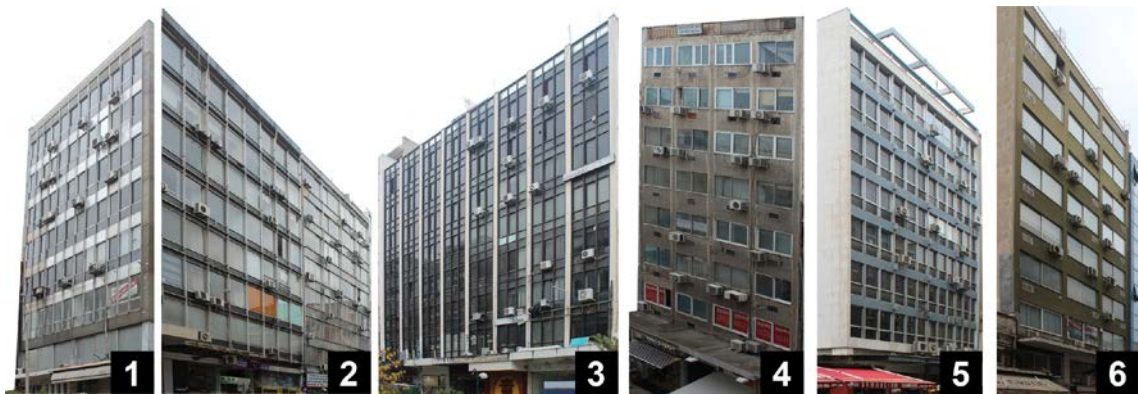
Figure 7: In this figure we see photos of the two types of buildings mentioned above. Buildings 1-3 are of curtain wall facade buildings, while buildings 4-6 are the more modernist repetitive windows type. The photographs were taken in the Central Business District (CBD) of Thessaloniki by the author.
