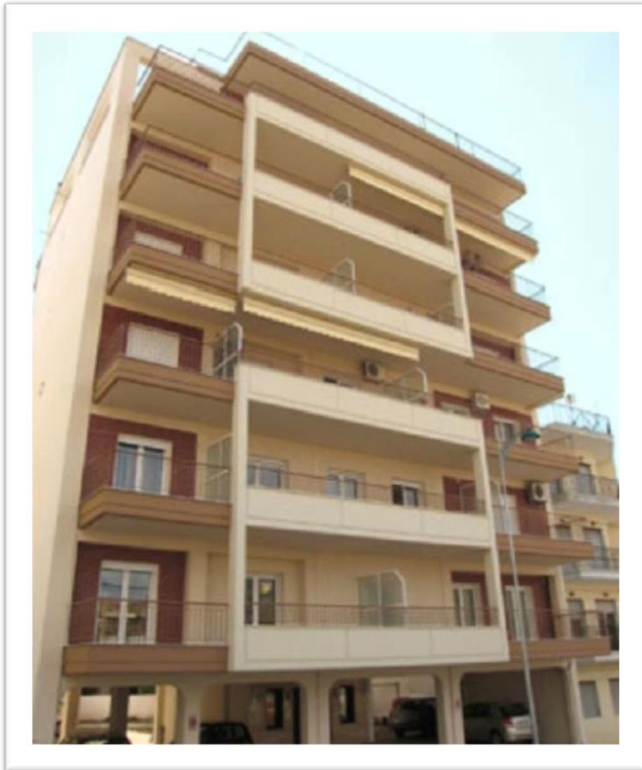
Figure 11: Typical MF building with Pilotis floor used as parking area [46]
