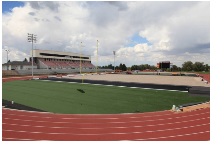
Figure 1: Southern Utah University Athletics Facility
