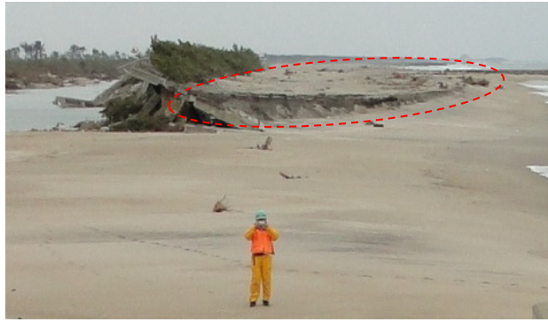
(a) Erosion of beach adjacent to the breaching at Yamamoto after the tsunami (cliff beach) (background: April 2, 2011)
