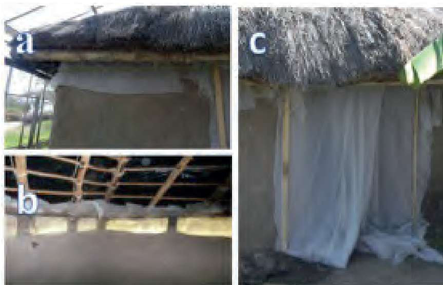
Figure 1. House screening applied for block-pull treatments. A visualizes how the eaves are screened and sealed off at the bottom by tying a rope around the wall of the house. B visualizes the eaves screening from inside the hut, as well as how additional gaps in the roof construction were sealed off using netting material. C visualizes the door screening with two overlapping layers of screening material that were nailed into the wall with slats.
