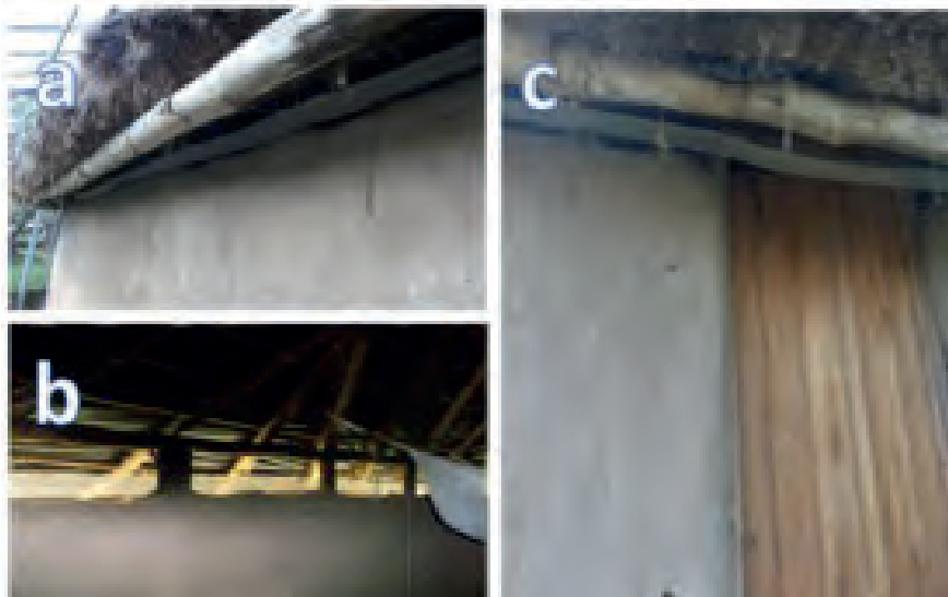
Figure 2. Band of cotton meshed netting material applied for push-pull treatments with dUDL repellent. A visualizes how the band is fixed around the eaves from the outside the house. B visualizes the cotton band from inside the hut. C visualizes how the band is fixed above the door.
