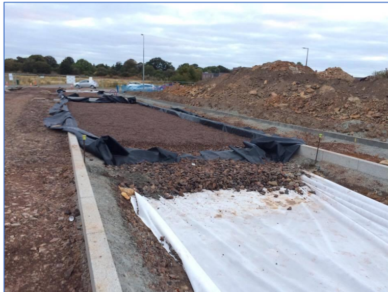
Fig. (6) Construction of permeable pavement [16].
