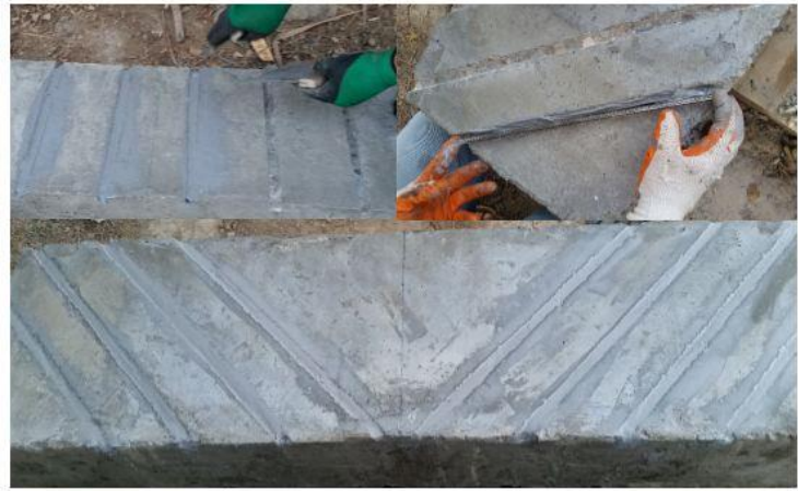
Figure (4) Imbedded Bars into Grooves
