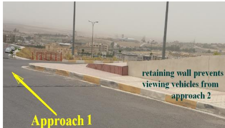
Figure (5) Retaining wall shorten the stopping site distance for vehicles at approach1
