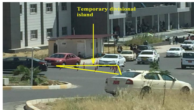
Figure (14) Temporary divisional island at entrance of approach 3
