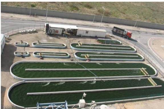
Fig 3: An aerial view of HRAP
