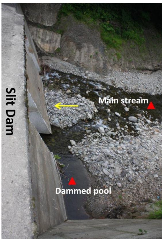
Figure 7.2 Observation points on the main stream and dammed pool at reach upstream of slit check dam of Wasada stream.
