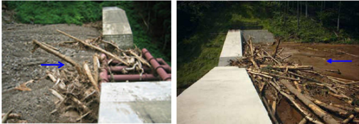
Figure 8.2 Debris flow and driftwood capture, left: at Hukui Pref., Japan, 1994, right: at Nagano Pref., Japan, 2006)
