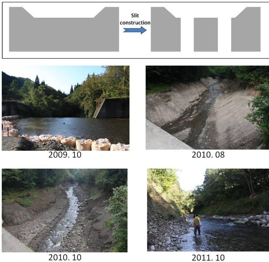
Figure 6.1 Slit check dam construction and landscape changes in Wasada stream
