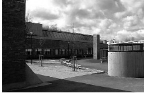
Pictures showing the main building before and after retrofit. Most visible features are the new daylight openings on the roof and new façades. The air inlet tower and a heat recovery unit (roof top) can be seen in the picture to the right. Architects for retrofitting: Hus Arkitekter AS. Photo left: B. Matusiak. Photo right: J. Rollan.
