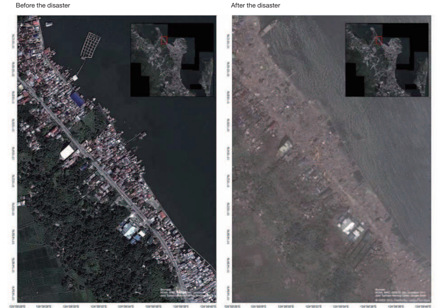
Tacloban was hit by a storm surge of 6 m. Houses along the seaside were swept away and aquaculture racks and piers were destroyed. (Mas, E and B. Adriano, IRIDeS Fact-finding missions to Philippines, pp.14, 2014.)
