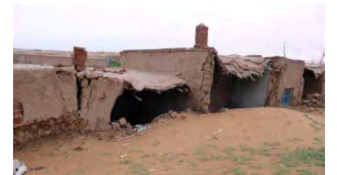
Fig.6 沙漠化で捨てられた家 Abandoned houses under the desertification in Inner Mongolia
