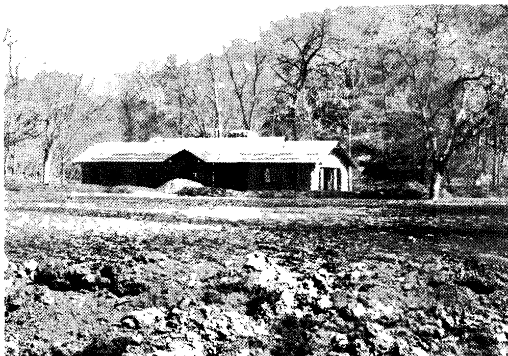
The main shelter house built in 1936 was totally submerged.
