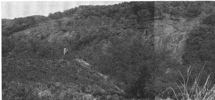
↑ Photo. 5 Failed zones at Nyuguchizawa.
