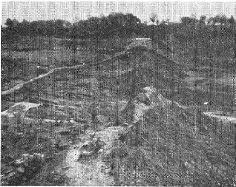
Photo. 8 Dam destruction of Hayakake-numa Reservoir
