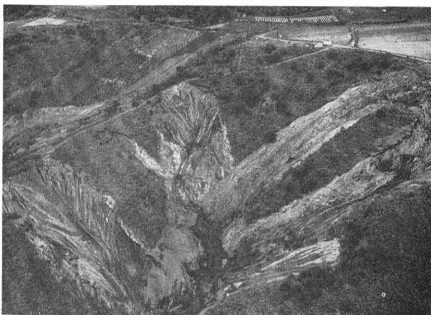
Photo. 1 Erosion areas and runways of six failed zones at Temmatai. Two erosion areas, the left and the right sides, are of Plane type and the central four erosion areas are of Scauper type.
