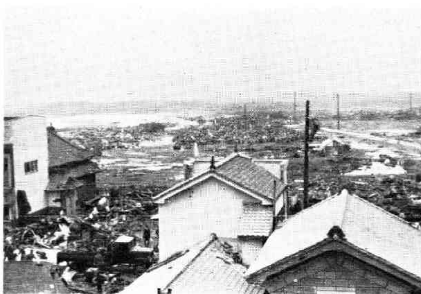
Photo. 6. Oofunado city was damaged severely by Tsunami.
