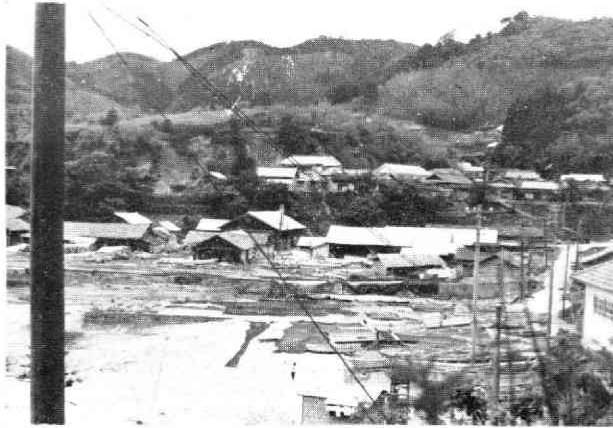
Photo. 10. At port of Ryori, the settlements once moved on high marine terrace were safe from the last Tsunami, whereas the houses located lower part were damaged by the Tsunami.
