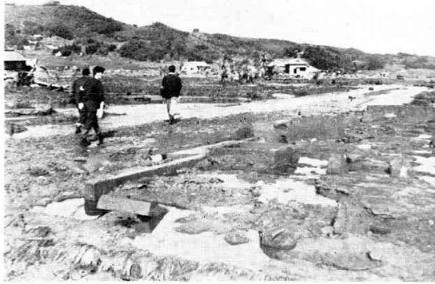
Photo. 3. At Ryogae located at the head of Hirota bay, settlers' houses were destroyed severely and their foundation-stones were only remained.
