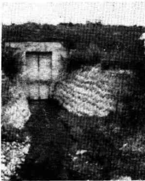
Fig. 3 Intake sluice-gate and ditch at the east bank of R. Omono.
