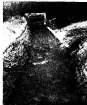
Fig. 6 Intake sluice-gate (4) of the Oirimizu canal in the upstream of R. Matsu.
