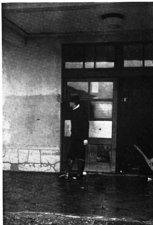
Photo. 10. Water height (about 4 m) is shown by the mark left by tsunami on the wall of Onagawa Station.
